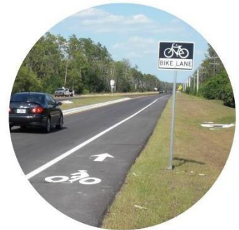
Paved Shoulder: a dedicated lane that is contiguous with the adjacent lane.
