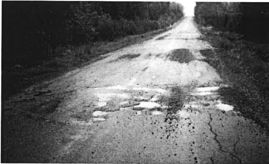
◀ Potholes from frost damage. Reconstruct.
