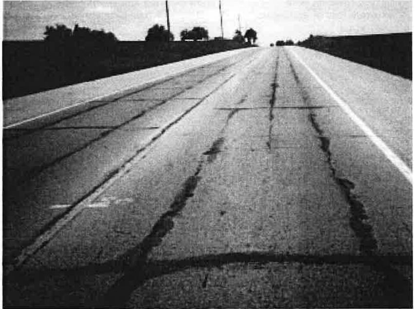
▶ Many wide and raveled cracks indicate need for milling and overlay.
