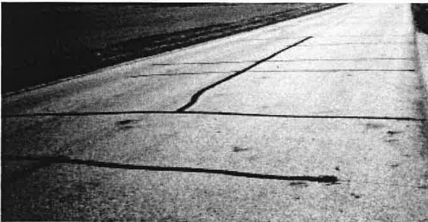
▼ Open crack, 1/2" wide; adjoining pavement sound.
