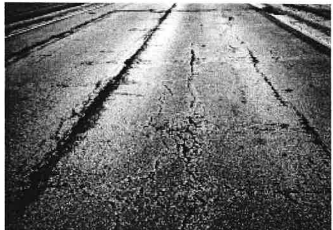
▼ Multiple open cracks at center line, wheelpaths and lane center.
