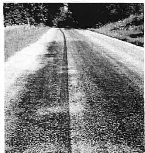
▼ Moderate flushing.
