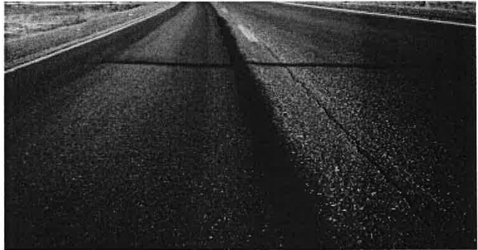
▶ Many wide and raveled cracks indicate need for milling and overlay.
