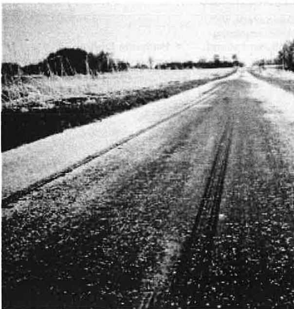
▼ Severe flushing.
