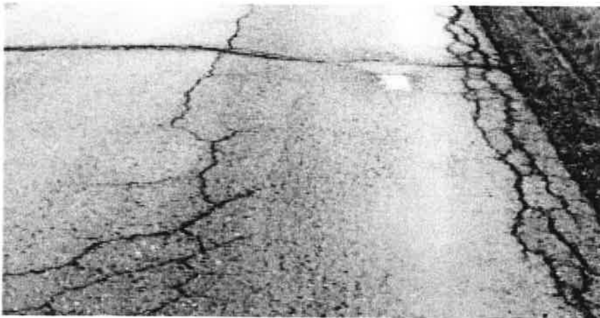
▶ First stage of wheelpath cracking caused by heavy traffic loads.
