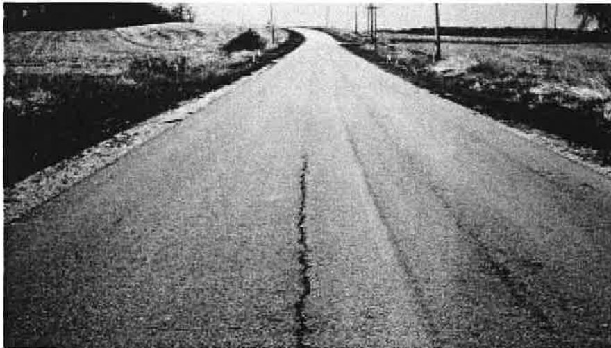
▼ Slight rutting; patch in good condition.
