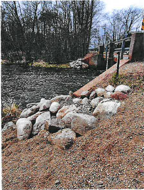
Dam wing walls
