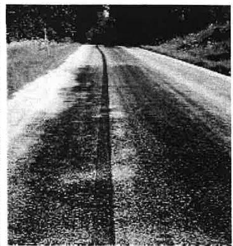
▼ Moderate flushing.
