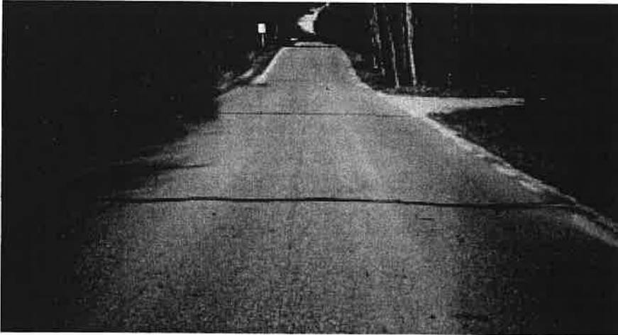
▼ Widely spaced, well-sealed cracks.
