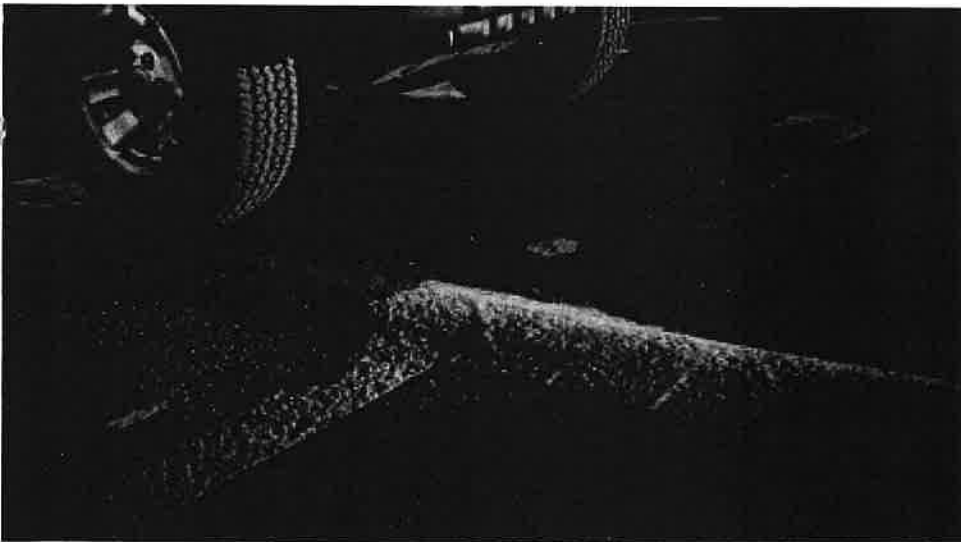
◀ Even slight rutting is evident after a rain.
