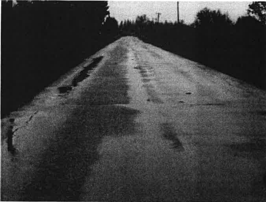
◀ Even slight rutting is evident after a rain.
