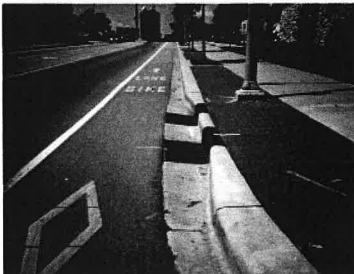
Urban drainage. RATING: Excellent
