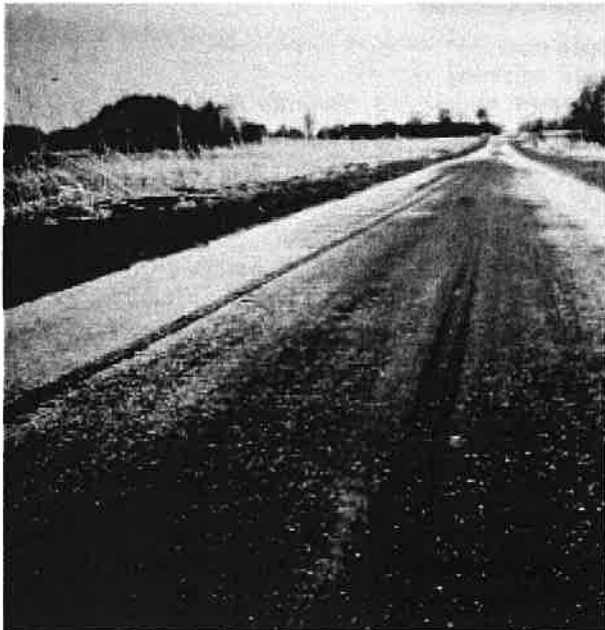
▼ Severe flushing.
