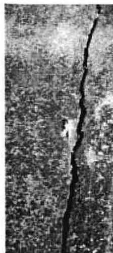
▼ Open crack, 1/2" wide; adjoining pavement sound.
