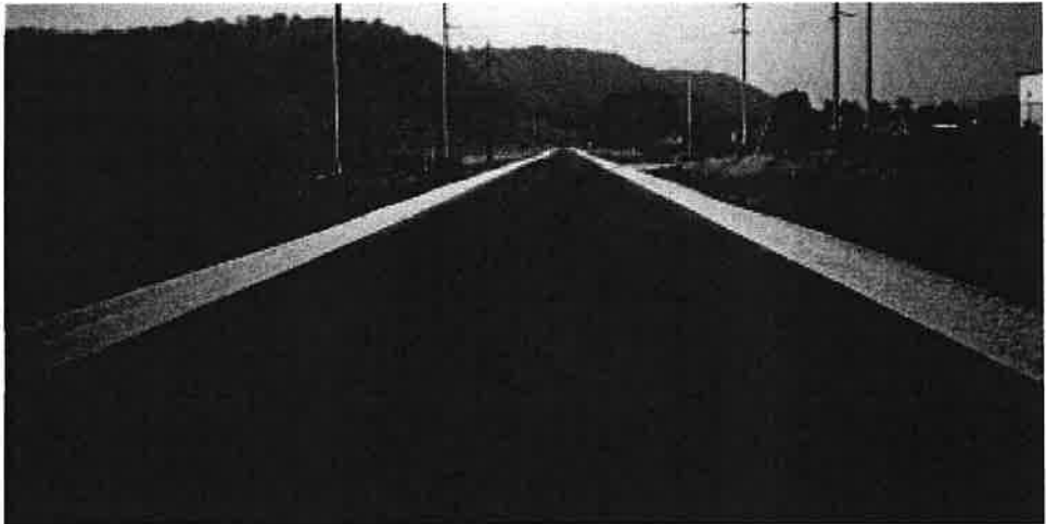
▶ RATING 9 Recent overlay, rural.
