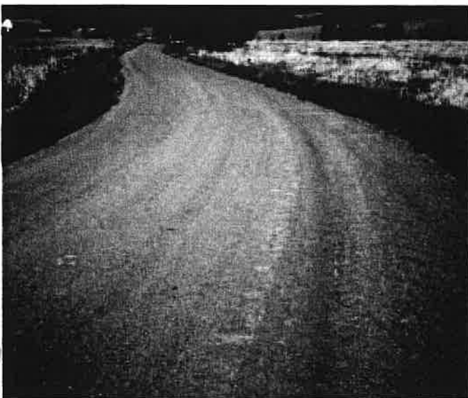
▲ New cold mix surface.
