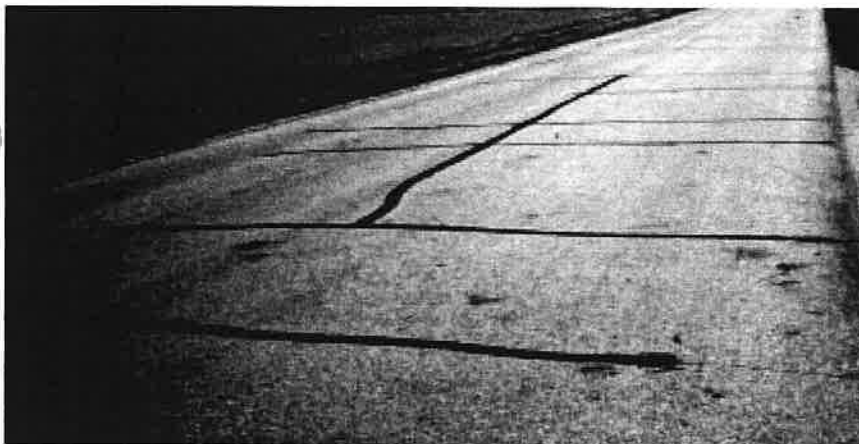
▼ Open crack, 1/2" wide; adjoining pavement sound.
